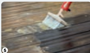
Apply NET-TROL® onto wet wood to neutralise.
