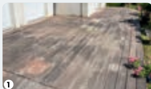
Initial situation: Darkened linseed oil + peeling red treatment + impregnated stain.
