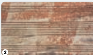
Initial situation: Darkened linseed oil + peeling red treatment + impregnated stain.
