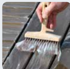
Apply NET-TROL® onto wet wood
